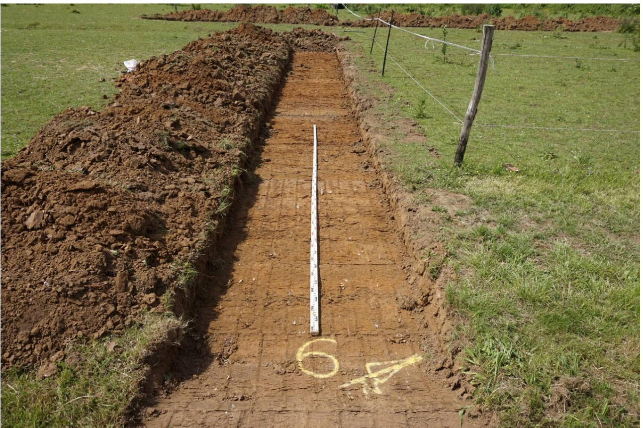
Plate 10: Looking west-north-west at Trench 6
